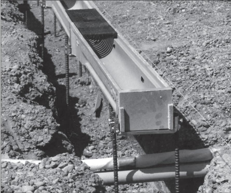
The POLYCAST® Installation Chair is the most efficient and economical means of setting a precast trench system. The installation chair supports the ends of the channels, aligns and locks the joint rigidly together and prevents the channels from floating. Adjusting channel elevation is easy with the POLYCAST® Installation Chair.
