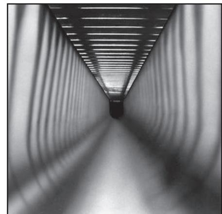
**ABOVE — Smooth interior finish of drain assures complete drainage**
